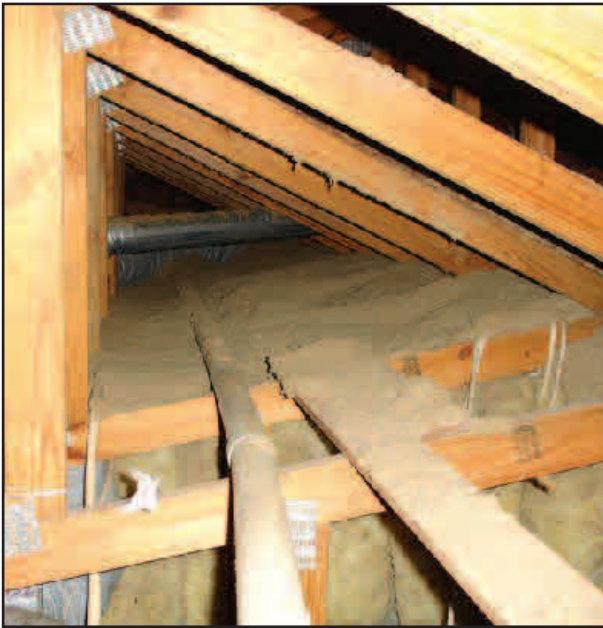
Figure 4 — The ac conduit parallels the antenna elements.
